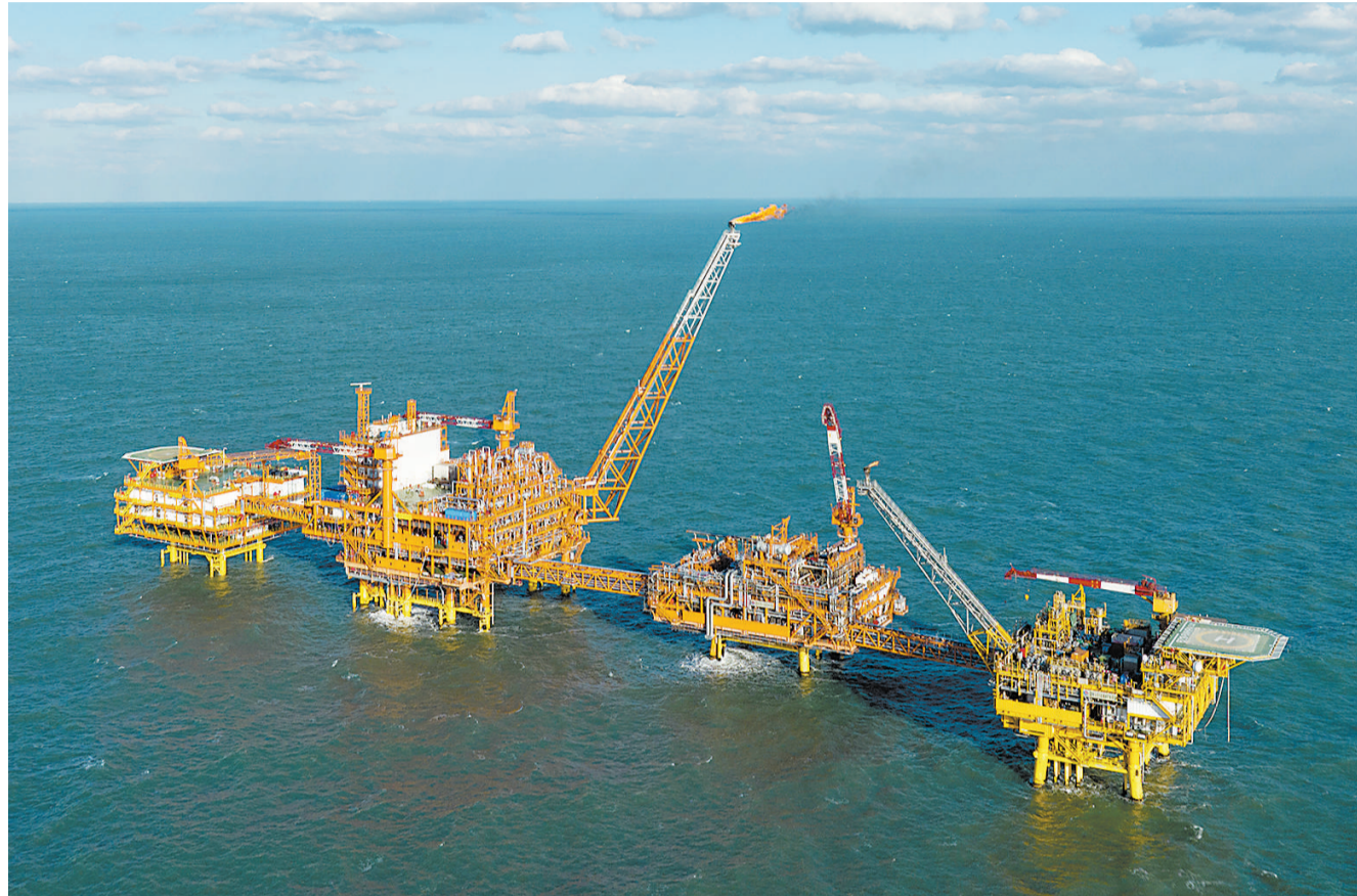
The Phase I project of Bozhong 19-6 Gasfield, the first 100 billion cubic meter gasfield in Bohai Sea, has been successfully put into operation, marking a new stage in the development of deep complex hydrocarbon reservoirs in China. (PHOTO: XINHUA)
